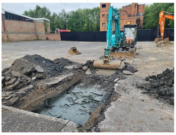
Plate 4 Removal of the overburden exposing natural clay alluvium, Trench 1, viewed from the northeast
